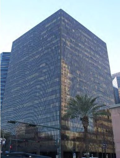
Orleans Tower Total Vacant: 80,286 SF Class B Built in 1977 No record of renovation
