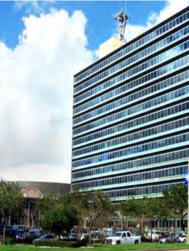
US Postal Total Vacant: 77,959 SF Class C Built in 1964 No record of renovation
