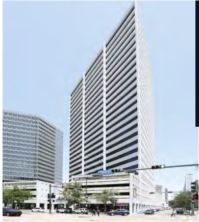
1515 Poydras St Total Vacant: 397,135 SF Class A Built in 1982 No record of renovation
